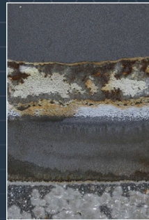
Complete coating failure of glass flake control system
